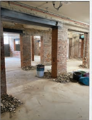
Plan A Commercial Interiors have begun stripping back the render to reveal the heritage brickwork, a feature of the fitout.
